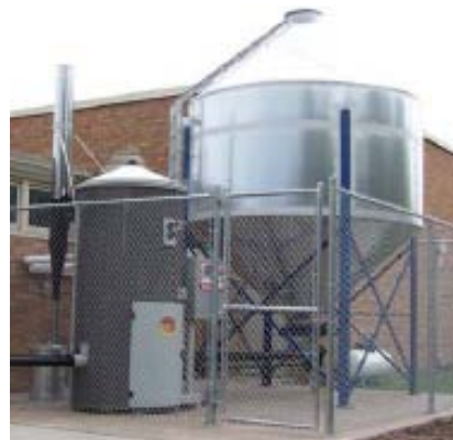
Figure 8. Biomass System
