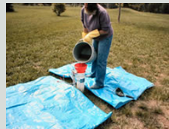
FIGURE 5 (POURING BLEACH SOLUTION IN WELL)
