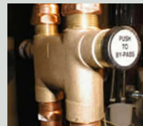
FIGURE 2 (BYPASS VALVES)
