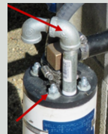
FIGURE 4 (VENT AND COMPRESSION BOLTS)
